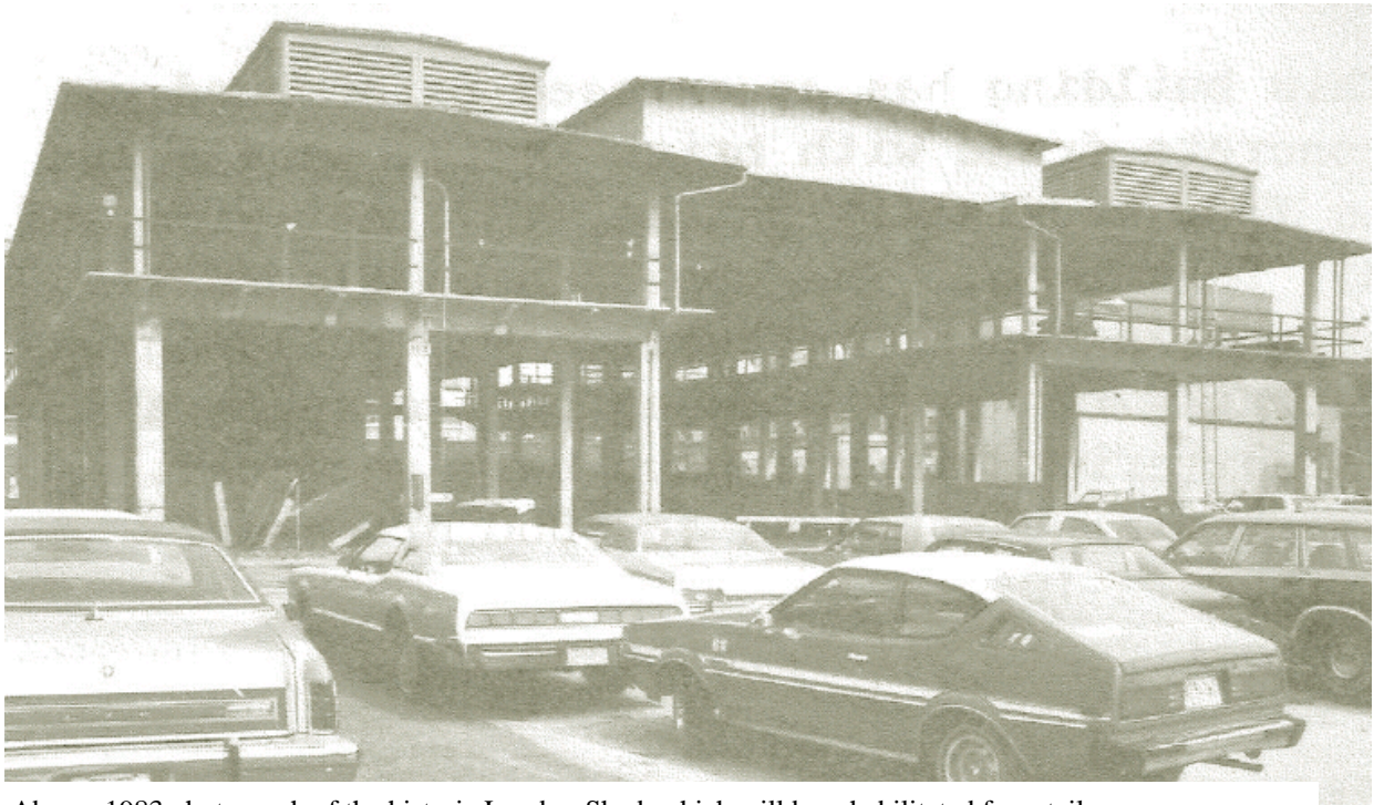
Above, 1983 photograph of the historic Lumber Shed, which will be rehabilitated for retail use.
